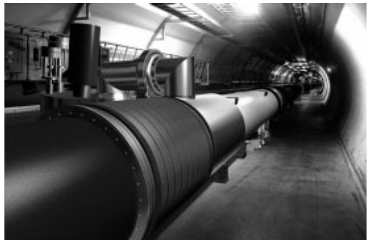
Figure 2: Simulated view of the LHC in its tunnel
